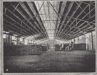
CORRUGATED IRON CONSTRUCTION INSURES GOOD PROTECTION FOR COFFEE AWAITING SHIPMENT 1—Front view of warehouse; 2—East view; 3—West view; 4—Interior of modern warehouse.
